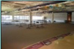
Open Work Area
